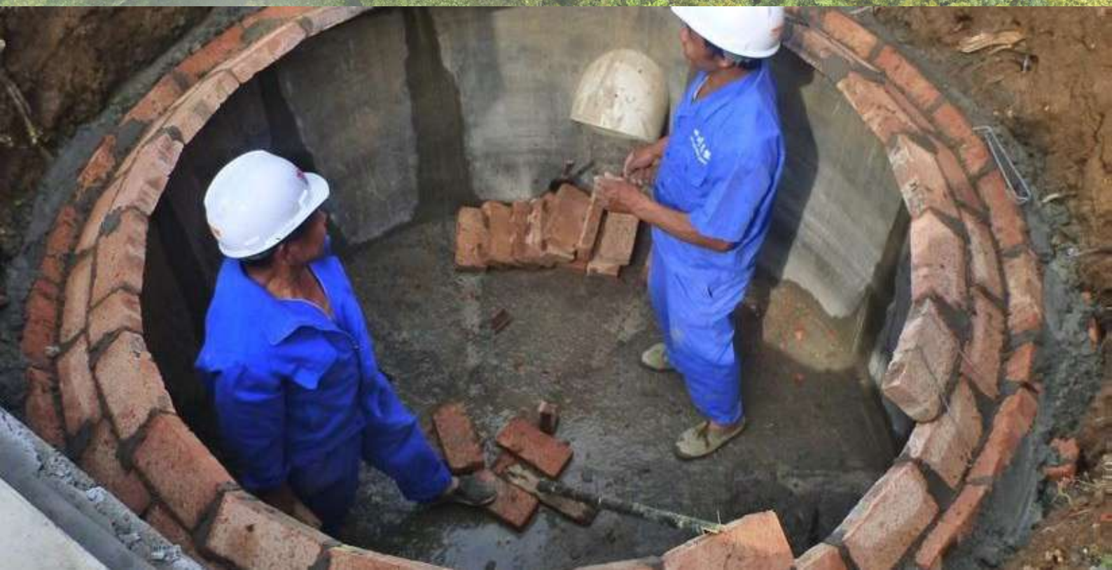
Sichuan Household Biogas Digesters, China
